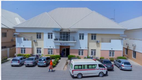
UMC Zhahir Hospital Kano, Nigeria
